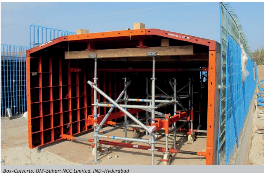
Box-Culverts, OM-Suvar; NCC Limited, IND-Hyderabad
