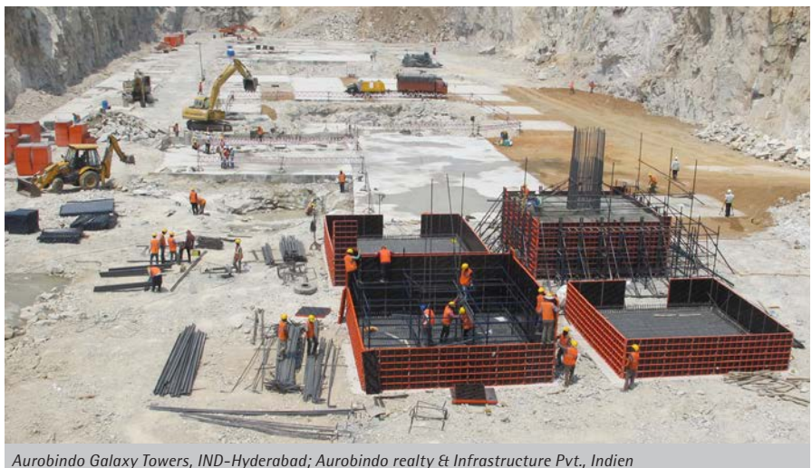
Aurobindo Galaxy Towers, IND-Hyderabad; Aurobindo realty & Infrastructure Pvt., Indien
